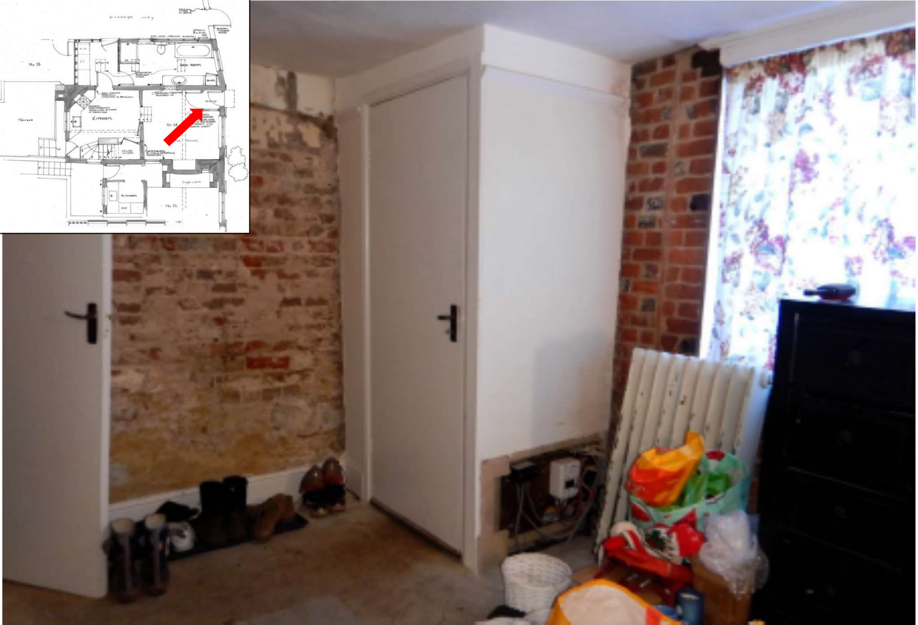
Figure 5: Plasterboard draft lobby to be replaced with an old oak joinery made draft lobby with leaded light side. Consumer unit (cpu) to be relocated within the rebuilt lobby.
